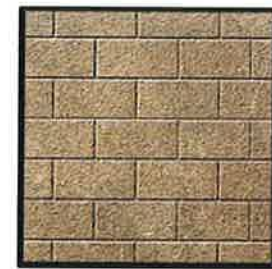
Split Face CMU (painted)
