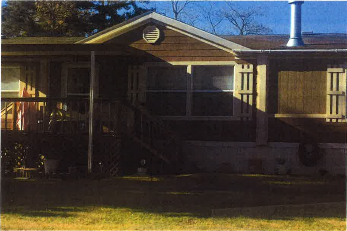
FRONT OF HOME SHOWING PORCH
