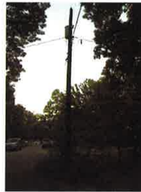
④ SITE PHOTOGRAPH SCALE: NTS
