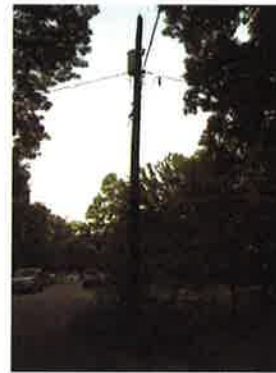
④ SITE PHOTOGRAPH SCALE: NTS
