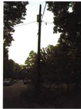
④ SITE PHOTOGRAPH SCALE: NTS
