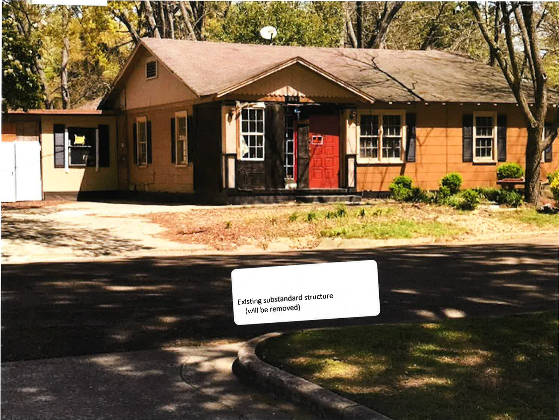
Attachment: 2019-035 ATTH 05 Photo of existing substandard structure (2061 : 2019-035 ORD rezoning
