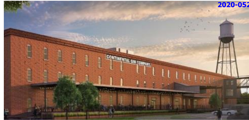
Continental Gin Building • City of Dallas Roofing • Glass/Glazing • Mechanical/HVAC • Lighting Solar • Ext. Walls • Elevators • Utilities • Assessment: $5M Annual Savings: 1.4M kWh; 11,000 mmBTU; 500 Kgal
