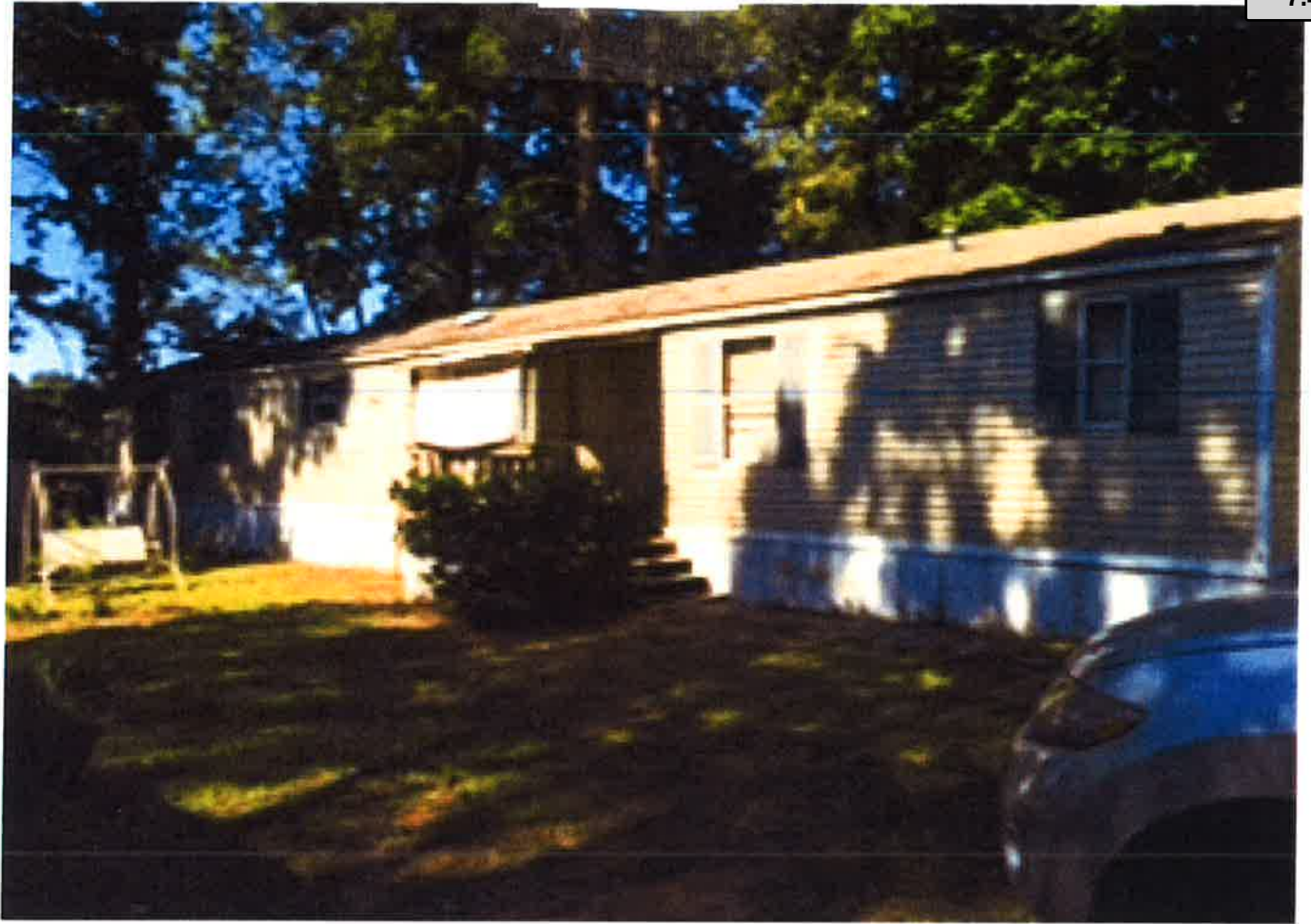
Attachment: 2016-084 ATTH 02 Photo of manufactured home (1512 : 2016-084 SUP for manufactured home at 2505 Phillips Lane)
