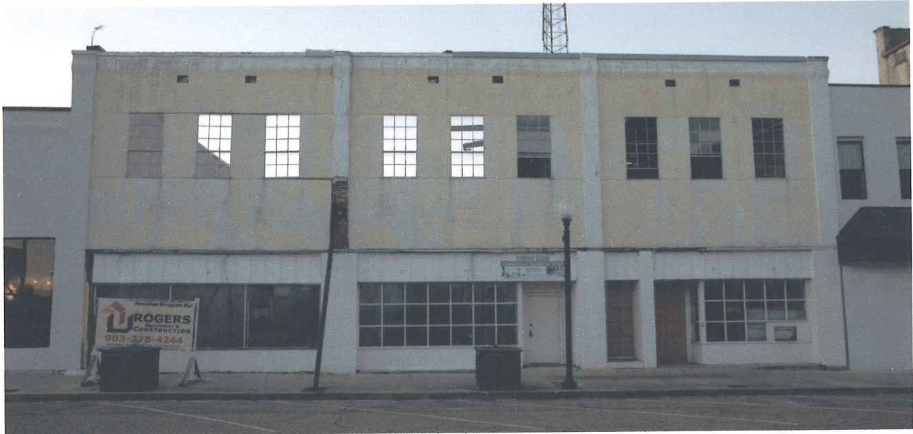
Current front façade.
