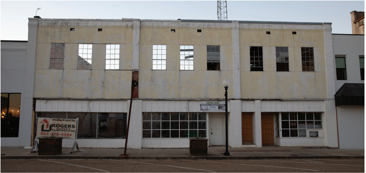
Current front façade.
