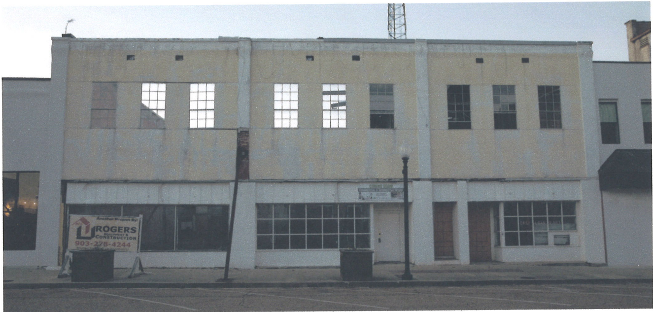
Current front façade.
